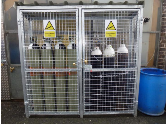
Fig. 10 – The gas cage. 4 x 50 litre air cylinders on the left, oxygen for nitrox on the right.
